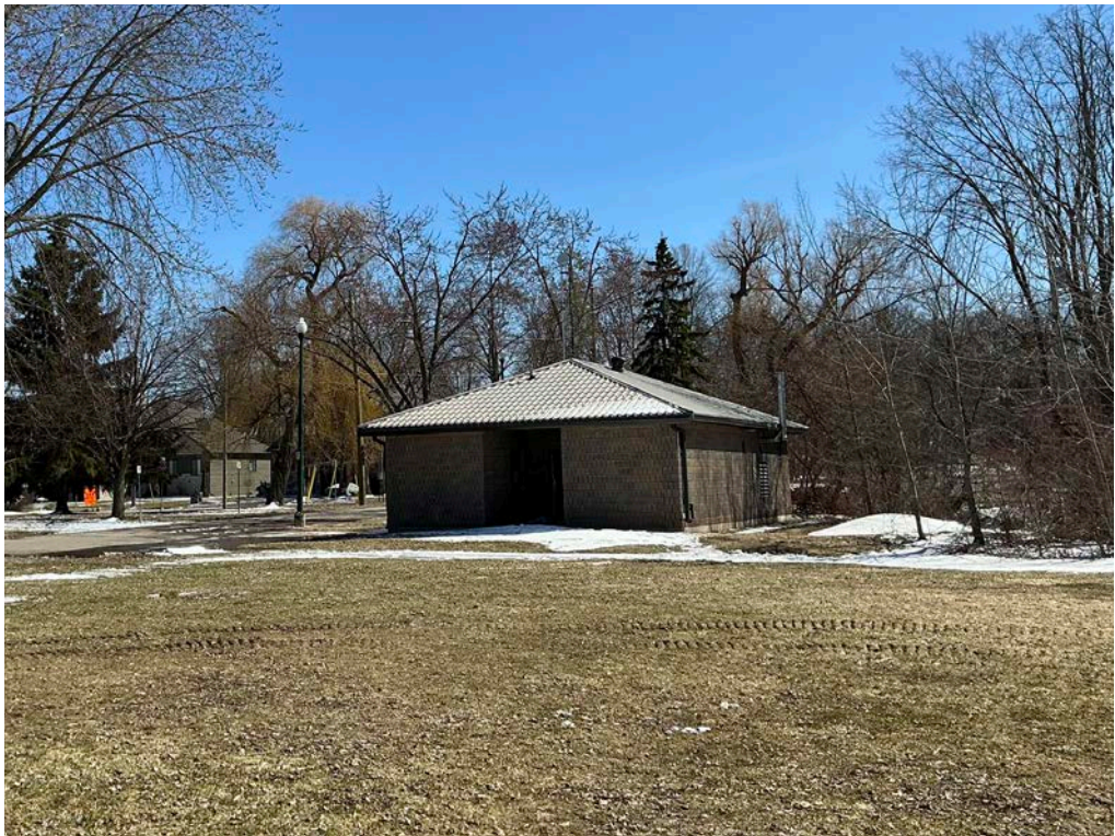
Existing washroom and pump station control building
