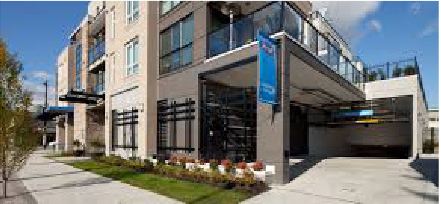
Discreet parking access from a side street. Credit:: Ventana Construction
