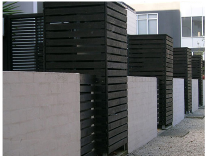
Screened waste and recycling enclosures.
