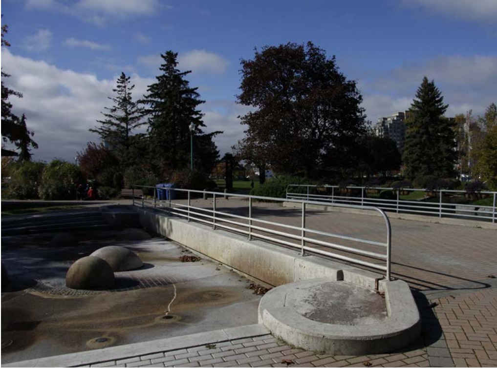
The north-west edge of the water feature area.
