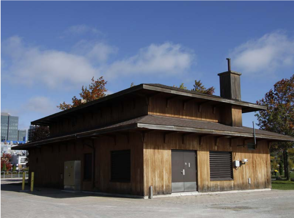
The washroom building at the west edge of the water feature area.
