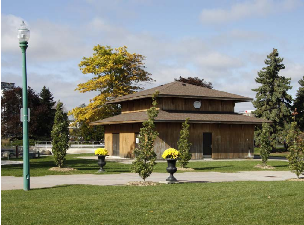
The pump house building at the north edge of the water feature area.
